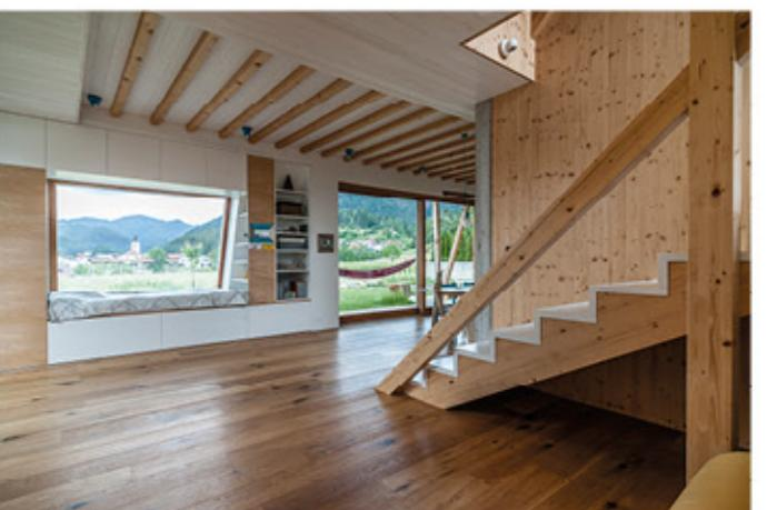
Prevladajoči element interjerja je vidna konstrukcija petih leseni trakov. Sodoben oblikovalski pristop in odprtost stavbe s fleksibilno in racionalno zasnovo dajeta hiši posebno prostorsko kakovost. | The interior is characterized by five exposed timber beams. The modern approach and open layout, with a flexible and rational basis, give this house its special spatial quality.
