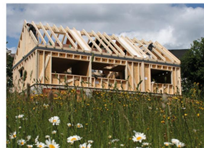
Pritličje je masivna opečna konstrukcija, nadstropje pa je izvedeno v leseni skeletni gradnji. | The ground floor is characterized by masonry, whereas the upper floor has been realized as a timber-frame structure.
